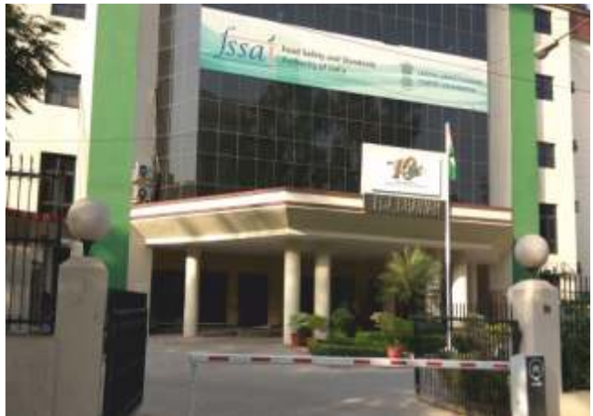
The newly renovated facade of FDA Bhawan where FSSAI is housed.
